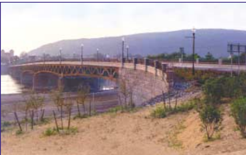
The Court Street Bridge replacement, located in Owego, NY, was a winner of the state's 2004 CSS Exemplary Project Award.
