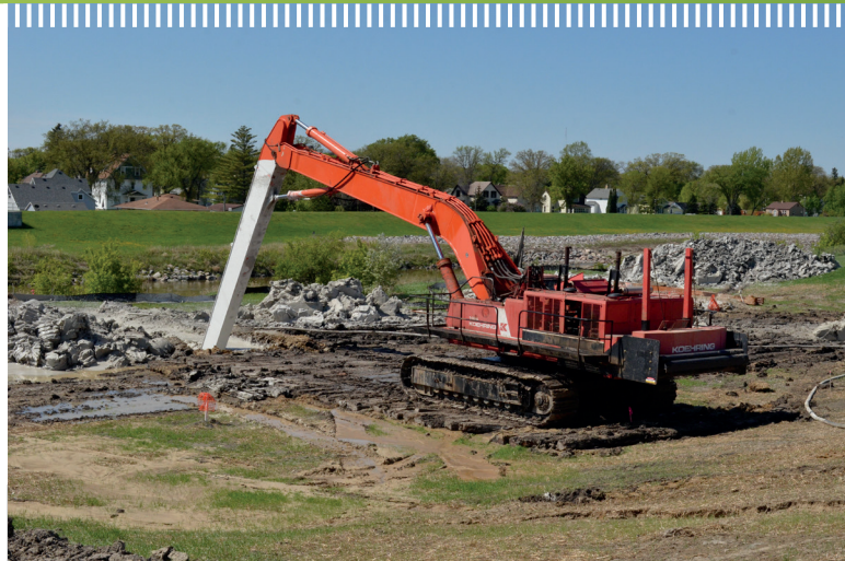
Excavation at Crookston Slope site. Photo: MnDOT
