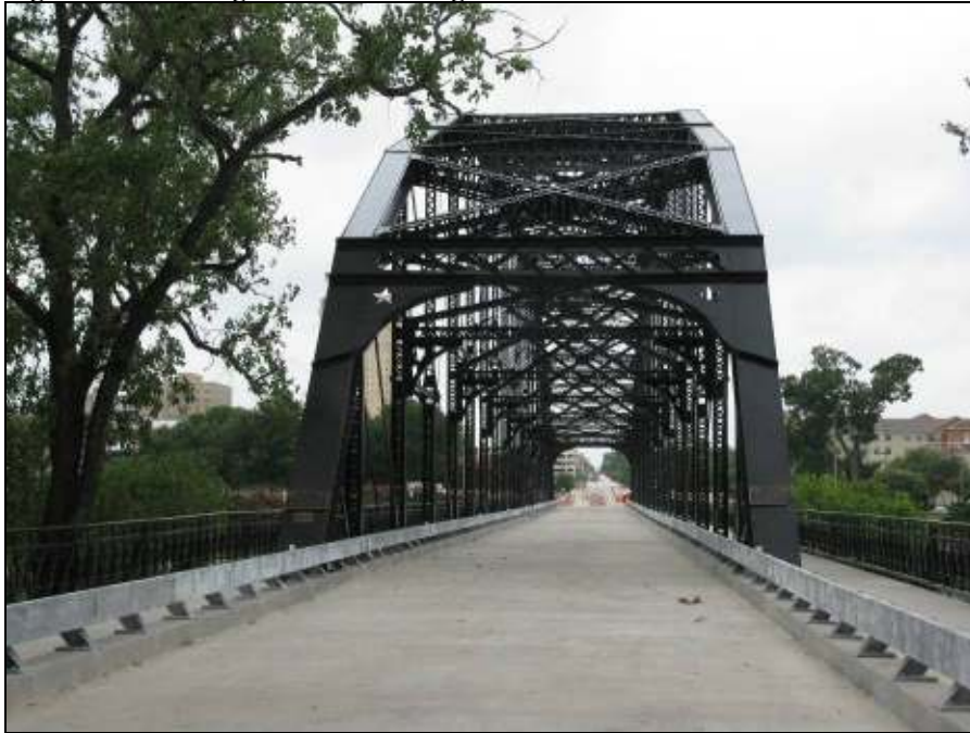
Figure 18. Washington Avenue Bridge
