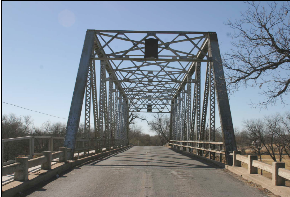
Figure 19. Lone Wolf Bridge
