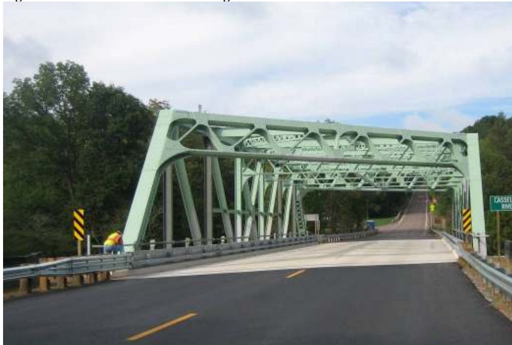
Figure 13. New Casselman River Bridge
