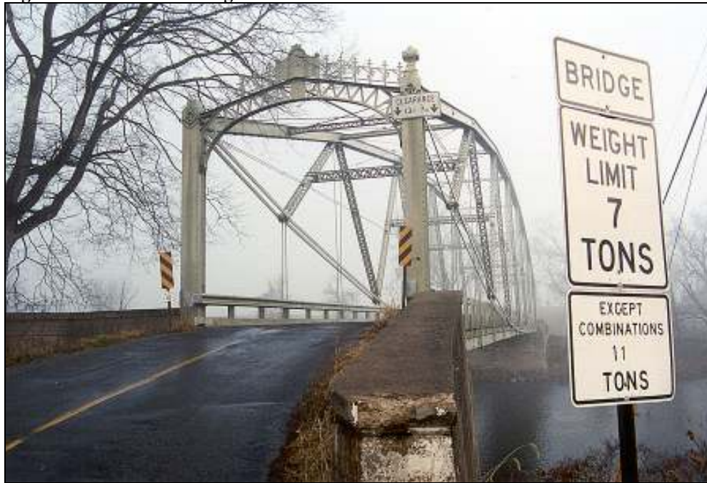
Figure 16. Pine Creek Bridge
