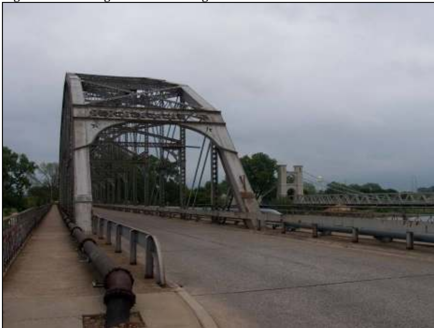
Figure 17. Washington Avenue Bridge
