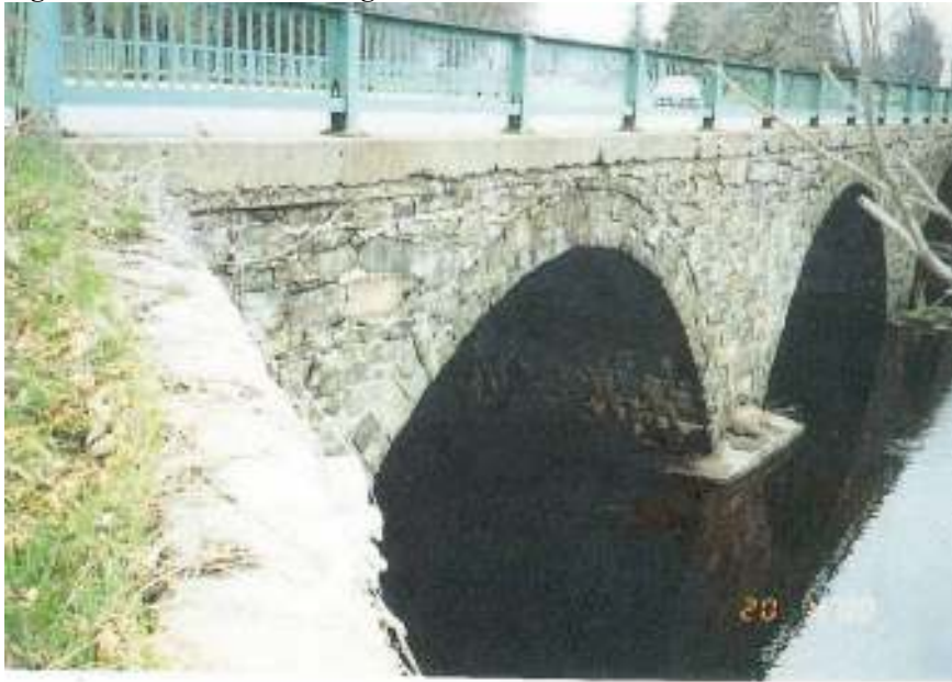
Figure 2. Prairie River Bridge
