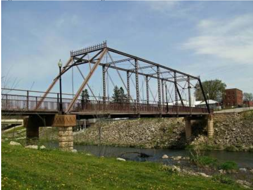
Figure 15. Walnut Street Bridge
