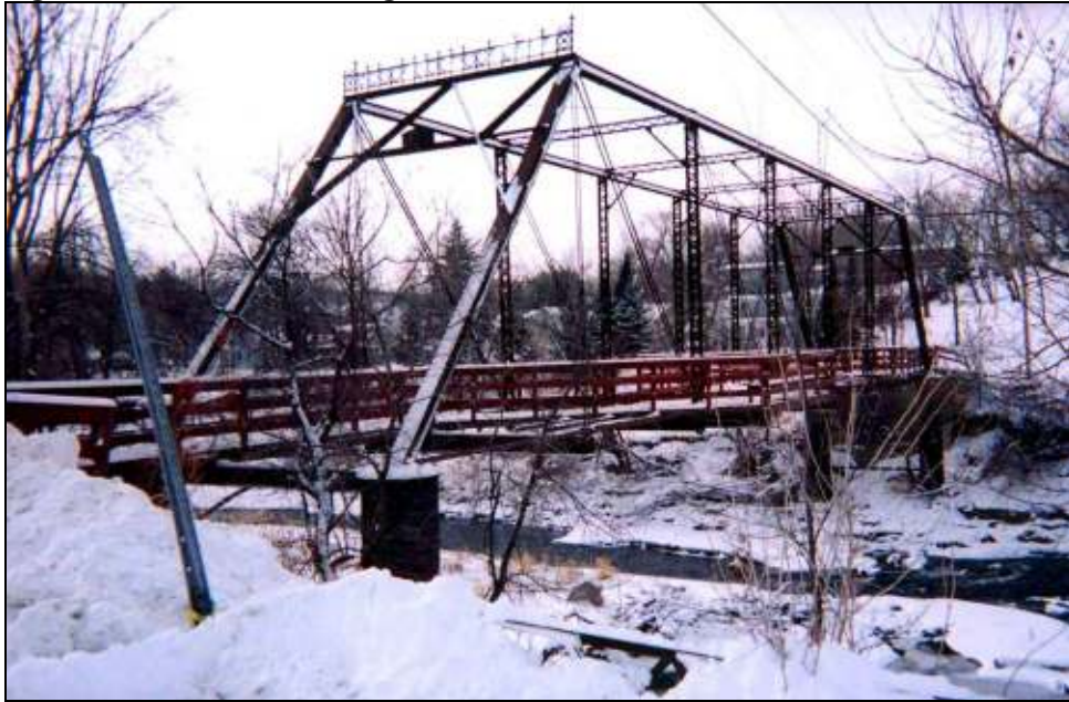
Figure 14. Walnut Street Bridge
