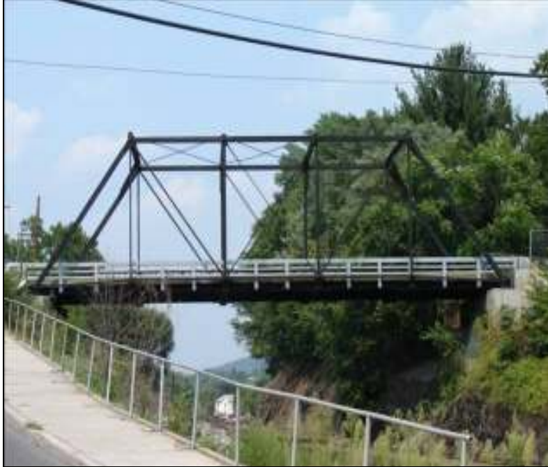
Figure 23. Hawthorne Street Bridge
