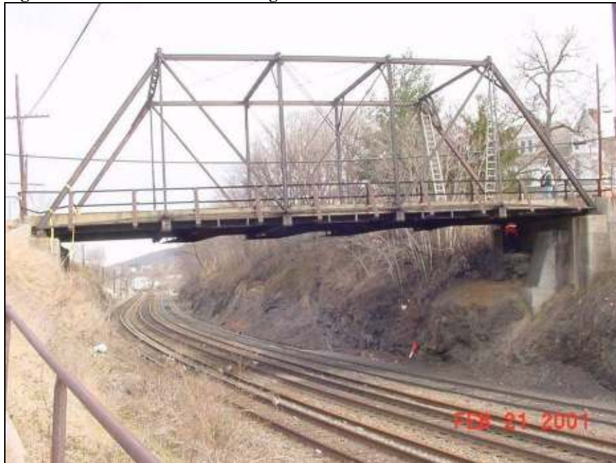
Figure 22. Hawthorne Street Bridge
