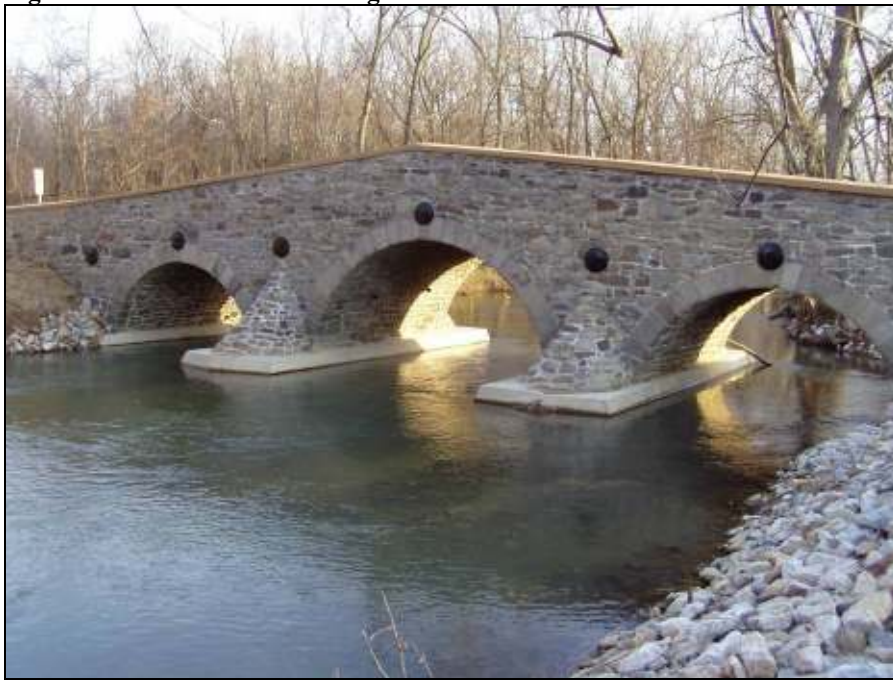
Figure 1. Johns Burnt Mill Bridge
