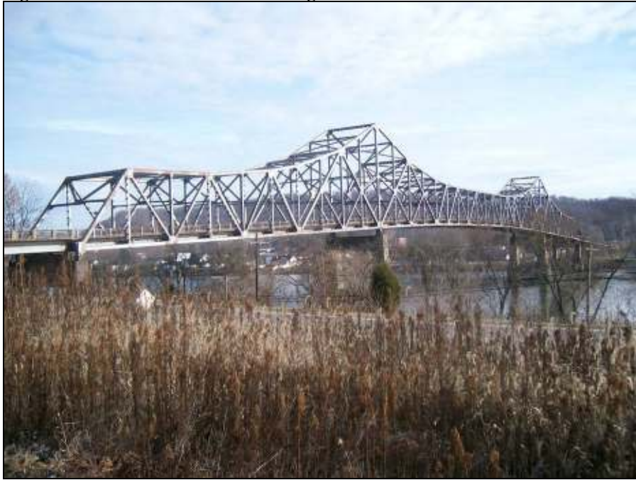
Figure 24. Ross Booth Memorial Bridge
