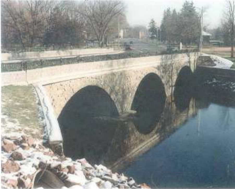
Figure 3. Prairie River Bridge
