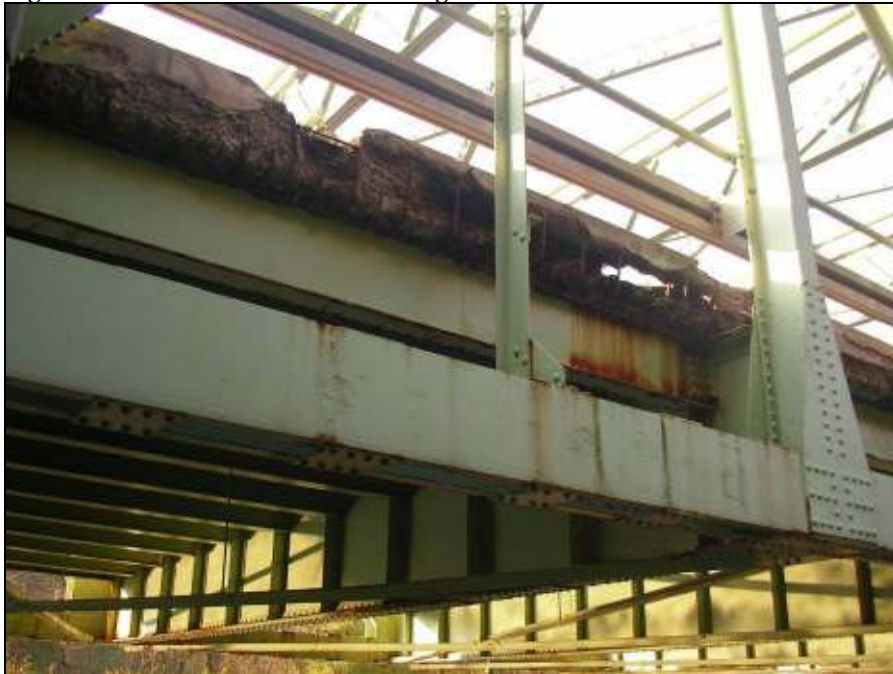
Figure 12. New Casselman River Bridge
