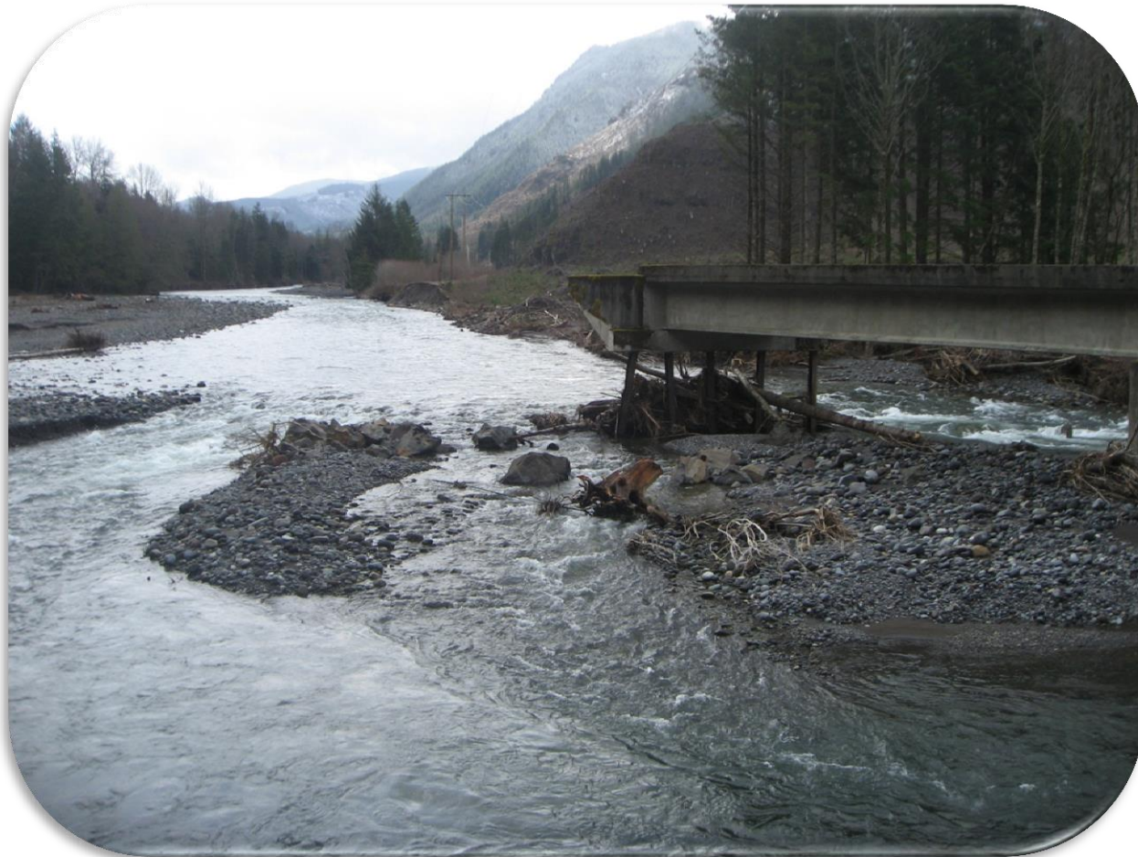
Scour and damage to structures - Just off SR410 White River
