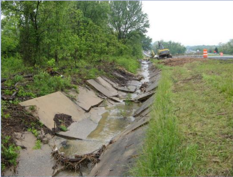
Removal of Concrete Channel at I 68 Partnership project with Watershed Group Planting by others USE III Stream
