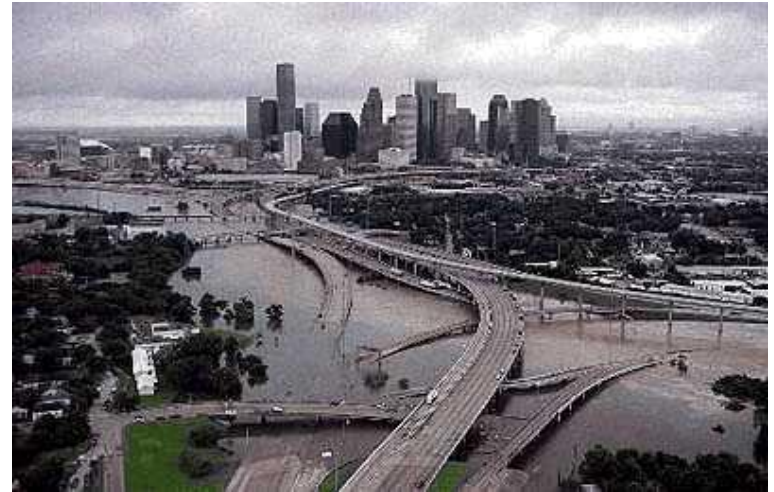
Flooded roadways in Houston
