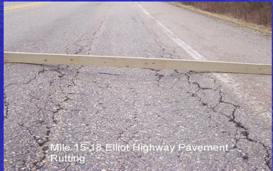
Alaska Highway Damage and rutting
