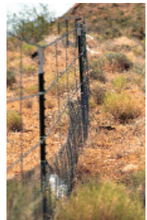
Specially designed barrier fences in California direct Desert Tortoises to storm-drain culverts that span the highway, and function as wildlife crossing structures for a variety of animals.
