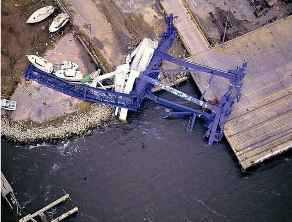
Columbus Street Terminal in Charleston, SC After Hurricane Hugo
