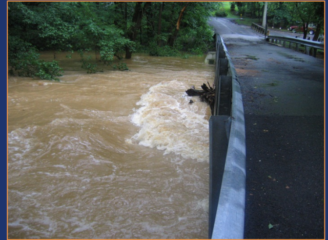
Floating Debris Lodged in a Bridge during Flood Event at Seneca Creek in Germantown, MD Photo Source: (FEMA/Skolnik 2006)
