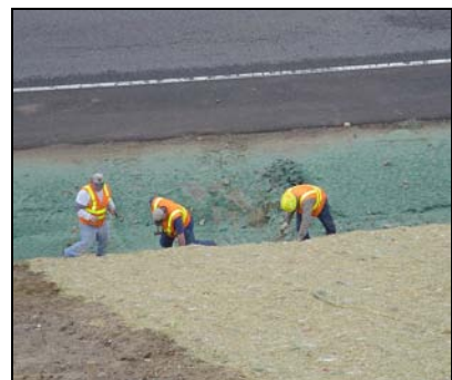
Straw matting and hydroseeding are effective erosion control measures.
