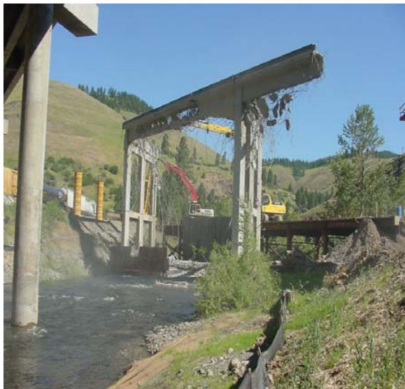
Demolition of old Quarry Bridges - courtesy of ODOT
