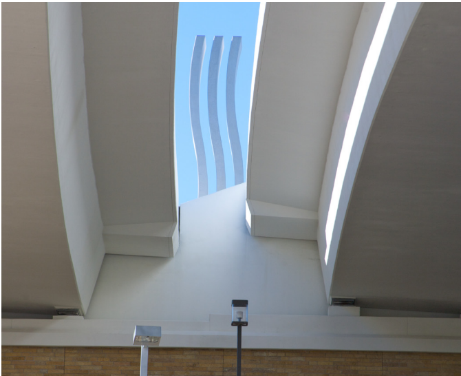
Curved gateway sculptures at each end of the bridge were developed with the VQAT. 30' tall precast panels representing the symbol for water are made of eco-friendly concrete with a nano-technology that cleans the air.
