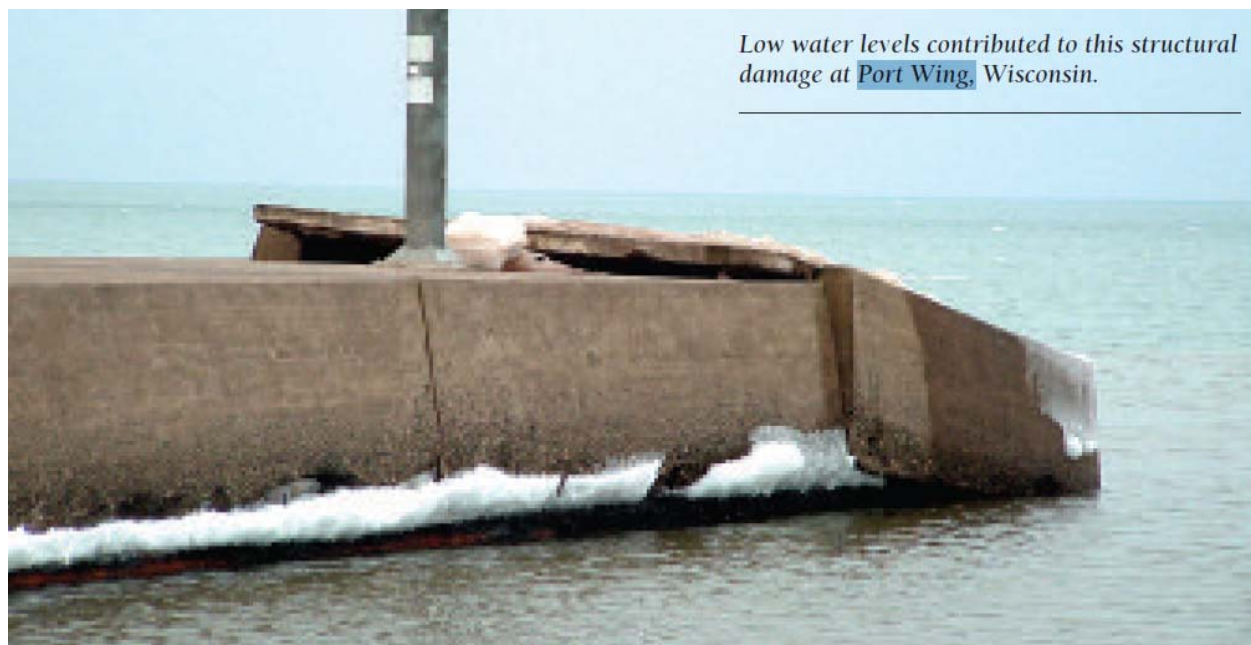
FIGURE 13: STRUCTURAL DAMAGE IN PORT WING, WI
